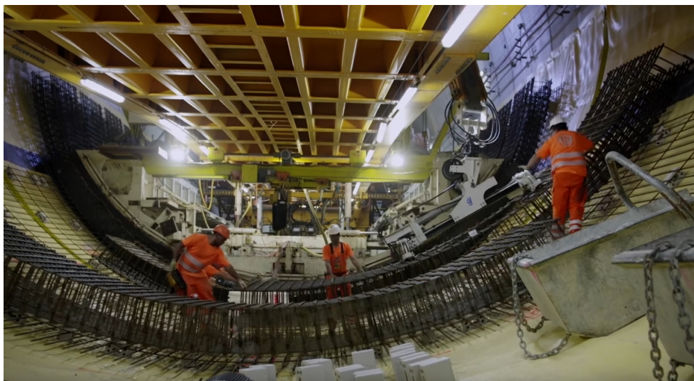
Figure 1.1.: Installation of the additional inner cast-in-place lining of the Sanierungstunnel Belchen with a thickness of 65 cm (Marti Gruppe, 2017).
