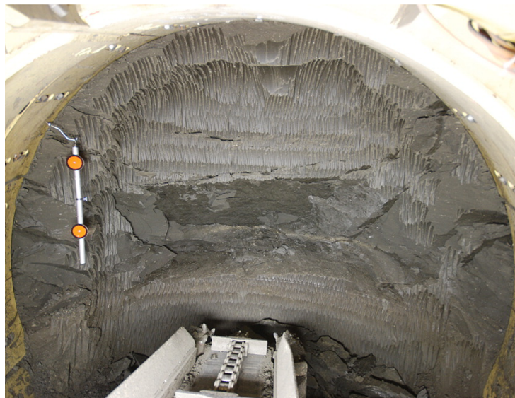
Figure 2.25.: Fractures observed on the excavation front (Praclay Gallery) at the HADES URF (Van Marcke and Bastiaens, 2010)
